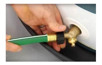
Some hose connections on new water heaters will require a screwdriver to open and close the water heater drain valve on the bottom of the tank.
